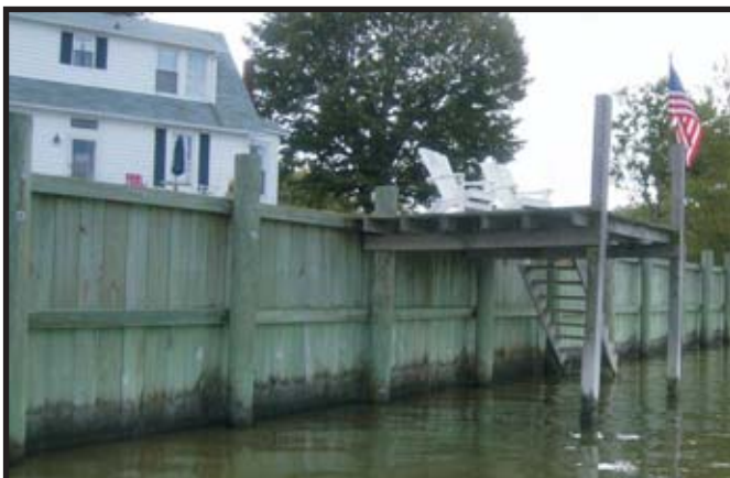
A bulkhead provides shore protection for houses, but it does not provide the land-water connection that is healthy for the Bay.
