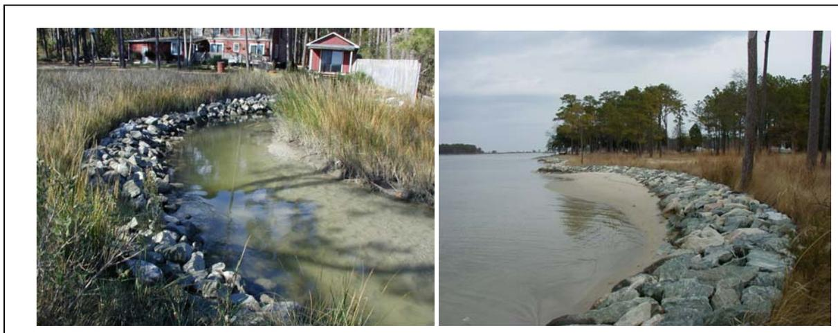
**Figure 5.** Unnecessary and inappropriate applications of marsh revetments are illustrated with these examples. The project on the left was located in a tidal channel and is excessive and unnecessary for erosion control (MA03). The project on the right was designed to perform like an upland revetment (LA07).
