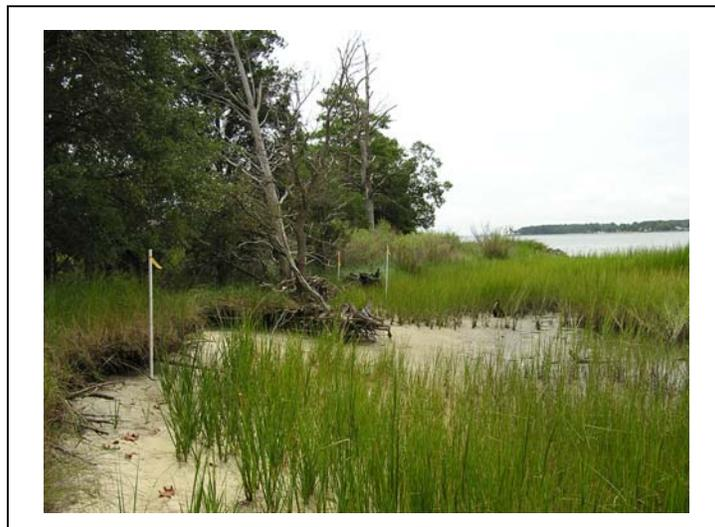
**Figure 6.** Spots of upland bank erosion were observed where the crest height of the marsh toe protection structure was less than +1 ft MHW in a medium energy setting. The white stakes indicate a proposed upland revetment (MA05). Raising the crest height of the marsh toe protection structure was encouraged instead to preserve the natural connections between the upland and wetland habitats.
