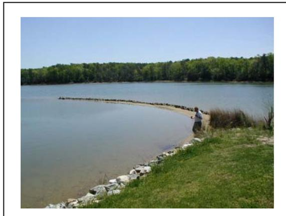
**Figure 8.** If upland revetments sever the landward end of a marsh spit, then marsh toe protection structures may not reverse the trend of “drowning” spit marshes. This is the only case where the revetment was not at all effective for erosion control (LA06).
