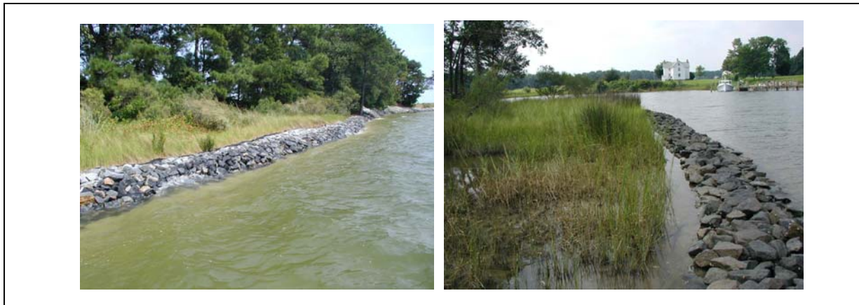
Figure 1. The two types of marsh revetments included in this study were “marsh toe revetments” placed directly against the edge of an eroding tidal marsh (left) and “marsh sills” offset from the edge of the marsh vegetation (right) or adjacent to non-vegetated intertidal area. Collectively, these rock revetments are referred to as “marsh revetments” for the purpose of this study.
