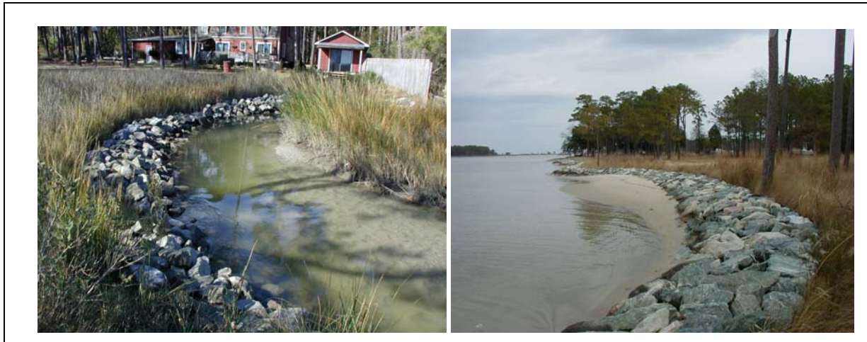
Figure 5. Unnecessary and inappropriate applications of marsh revetments are illustrated with these examples. The project on the left was located in a tidal channel and is excessive and unnecessary for erosion control (MA03). The project on the right was designed to perform like an upland revetment (LA07).
