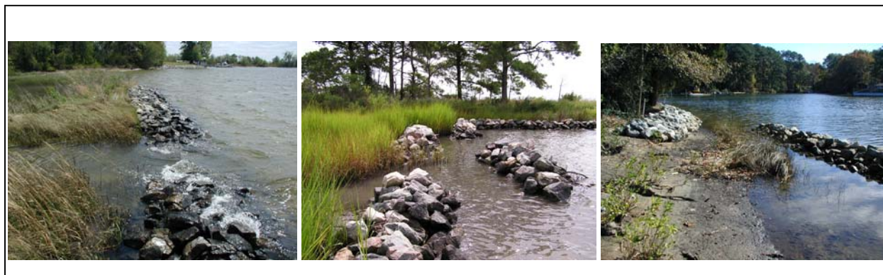
Figure 3. Three different types of tidal openings are illustrated, including a straight gap (left), offset gaps at a pocket marsh (center), and an end opening instead of tying into the upland bank or other erosion control structure (right).
