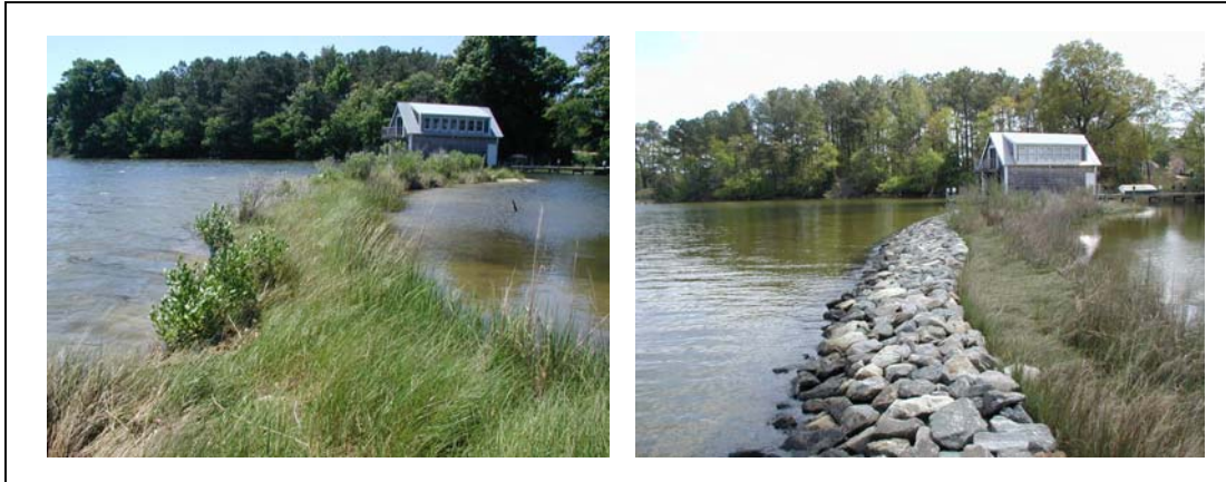
Figure 9. The placement of marsh toe protection structures along the entire length of marsh spits may adversely interrupt the sediment transport process that maintains suitable elevations for marsh vegetation. In this case, the revetment base width also seemed to be excessive (8 ft) compared to the width of the existing marsh (NU08).
